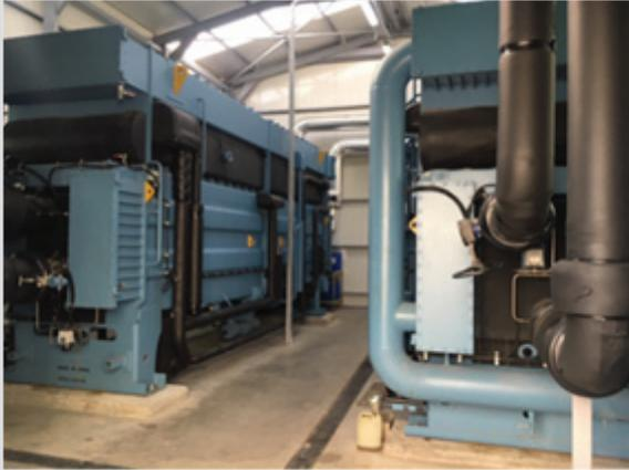
There was an estimation that after the “heat recovery project” at PE, steam generation would be reduced. In order to produce required amount of steam, two new hot water vam chiller machines have been bought to utilize the waste heat of the engines jacket water and Chips Plant column water. A new heat exchanger was installed at Chips Plant to utilize the heat of the vapors of the column to generate hot water to operate new vam chillers.
