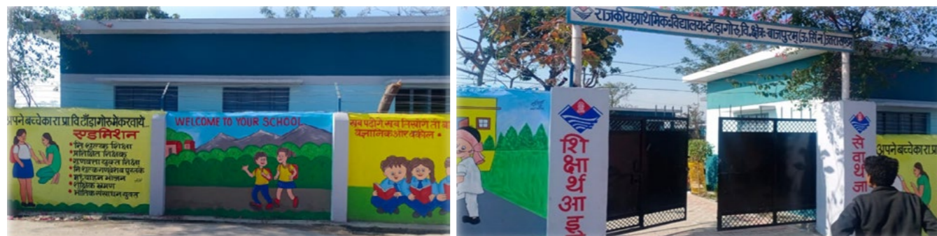
Renovation of Primary School Bazpur
